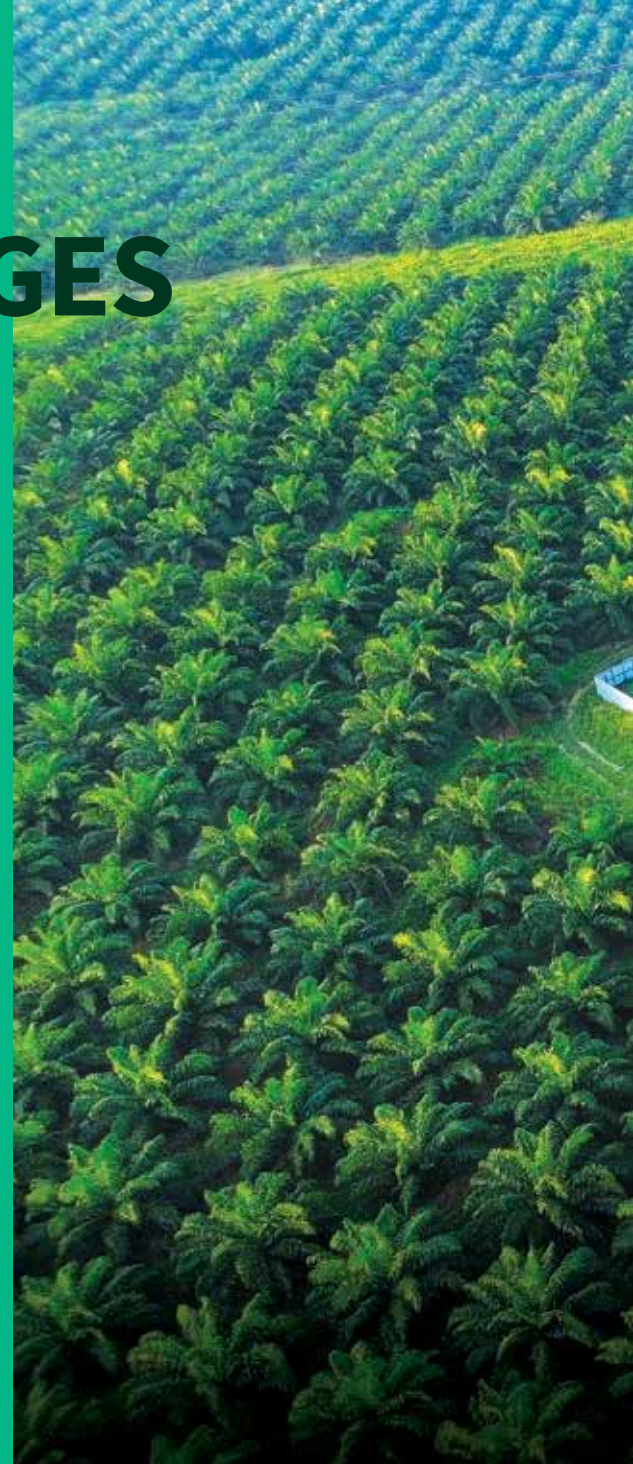
View of biogas plant at Telok Sengat Palm Oil Mill, Johor
