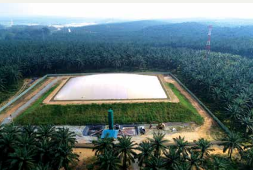
Biogas plant at Telok Sengat Palm Oil Mill
