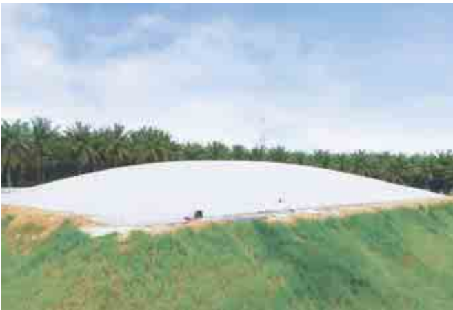
Lagoon biodigester system at our Biogas Plant, Telok Sengat Palm Oil Mill
